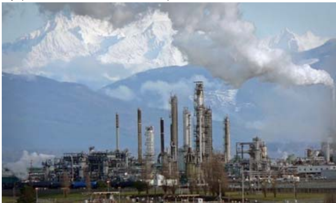
Figure 2. Tesoro Anacortes Refinery
